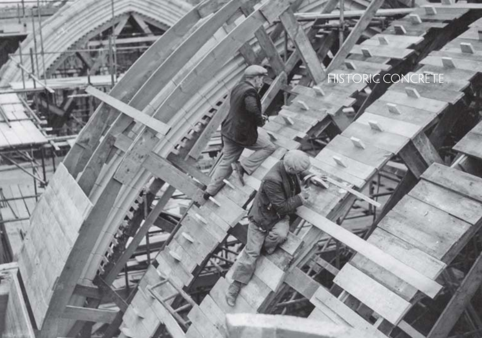
Creating formwork for the chancel arches in 1939. (Photo: Guildford Cathedral Archives.)
