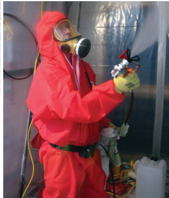
Asbestos removal in a sealed cabinet under the west gallery, May 2016.
