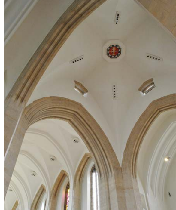
Crossing and quire ceilings after plaster removal.
