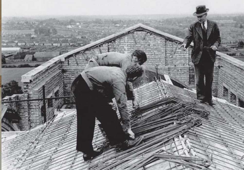
Fixing reinforcement for roof slab. (Photo: Guildford Cathedral Archives.)
